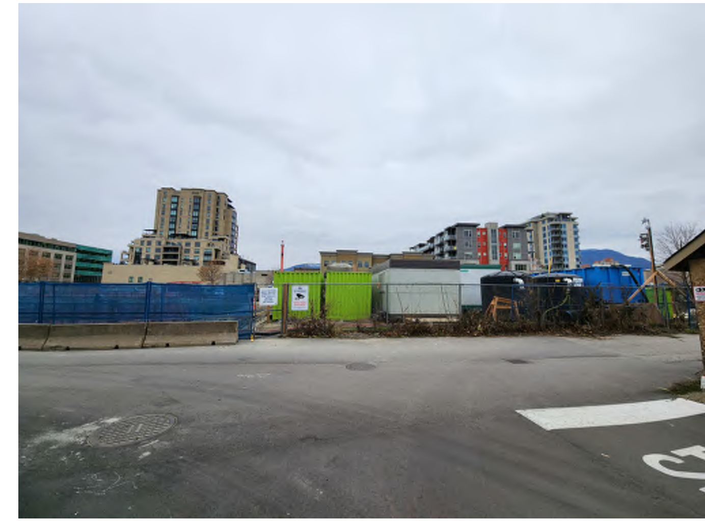
5. View facing West from the end of Fuller Ave
