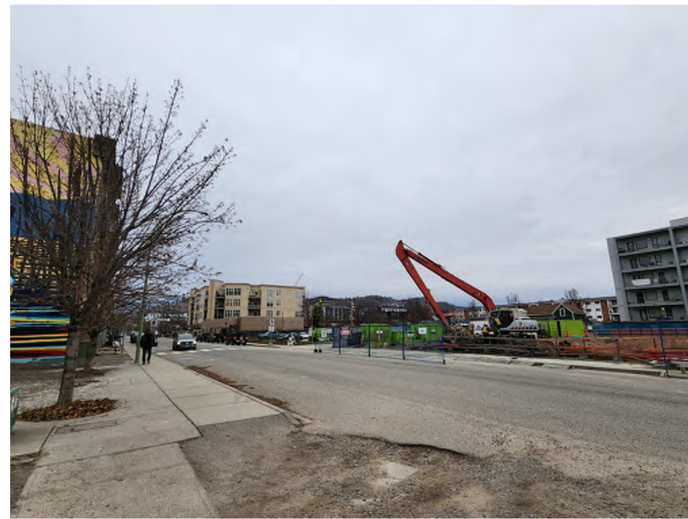
3. View facing North from the parking lot across UBCO downtown development
